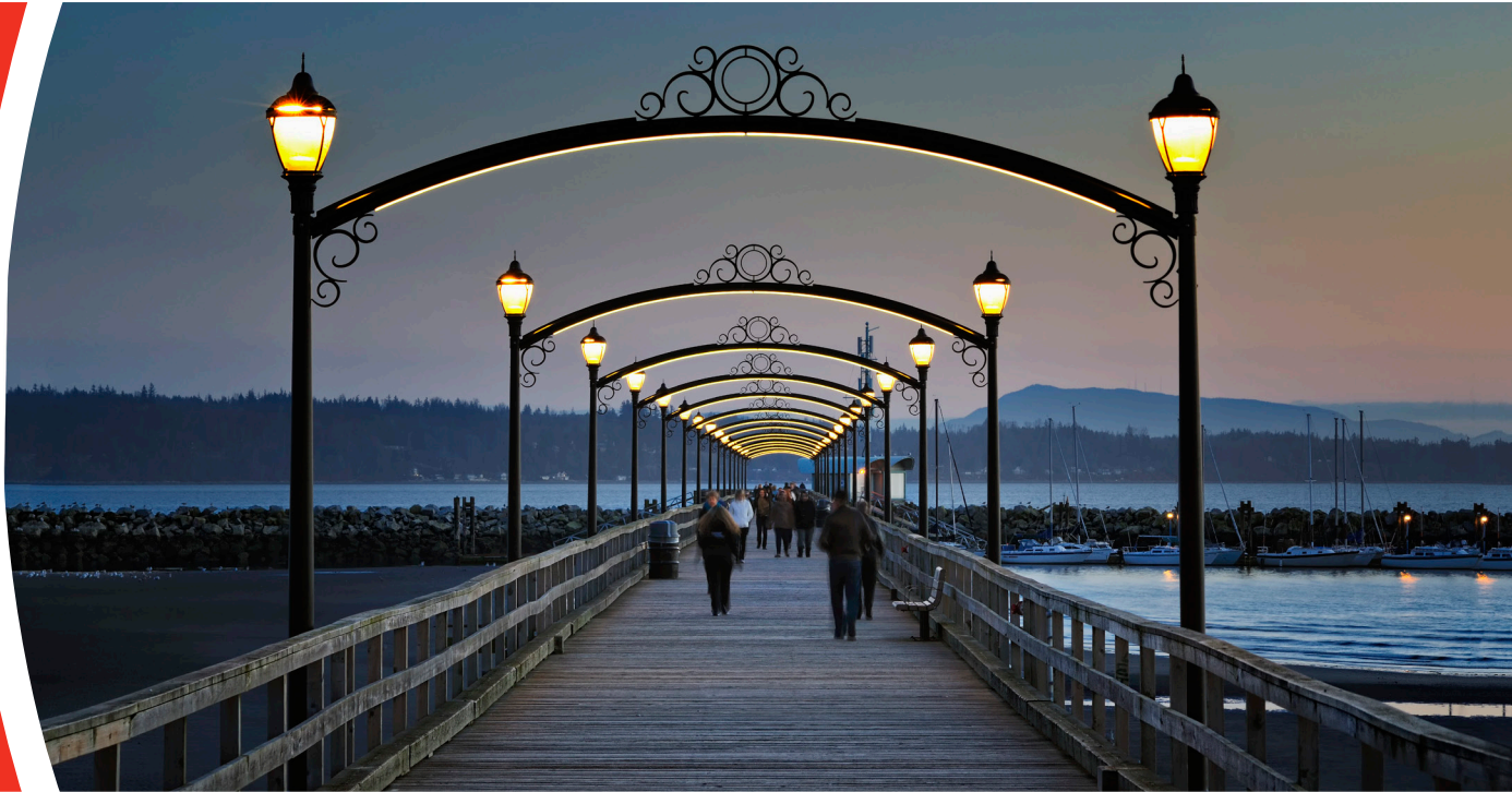
Spanning 1,500 feet, White Rock Pier features overhead arches edged with iLight Plexineon White 1X fixtures.
