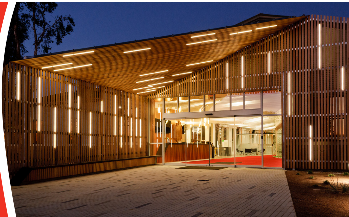
Vertical strips of Plexineon highlight the entrance to the new Claremont University Consortium (CUC) administrative center.
