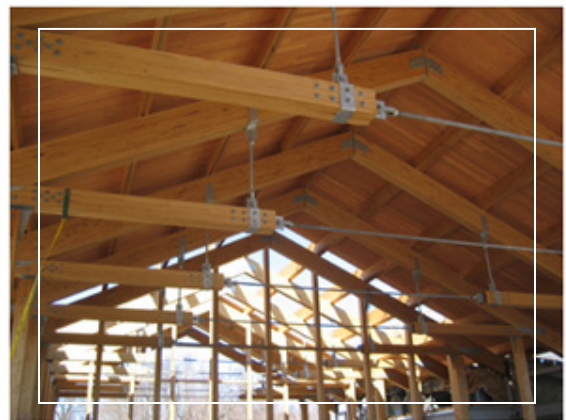
Ceiling view of the Lower School multipurpose room
